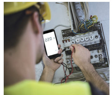
Electric Power Inspection
